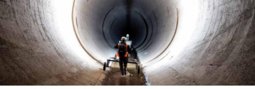
Workers use 3D LiDAR to survey the 20-foot-wide, 25,000-foot-long Carley V. Porter tunnel, a key part of the State Water Project in Kern County.
