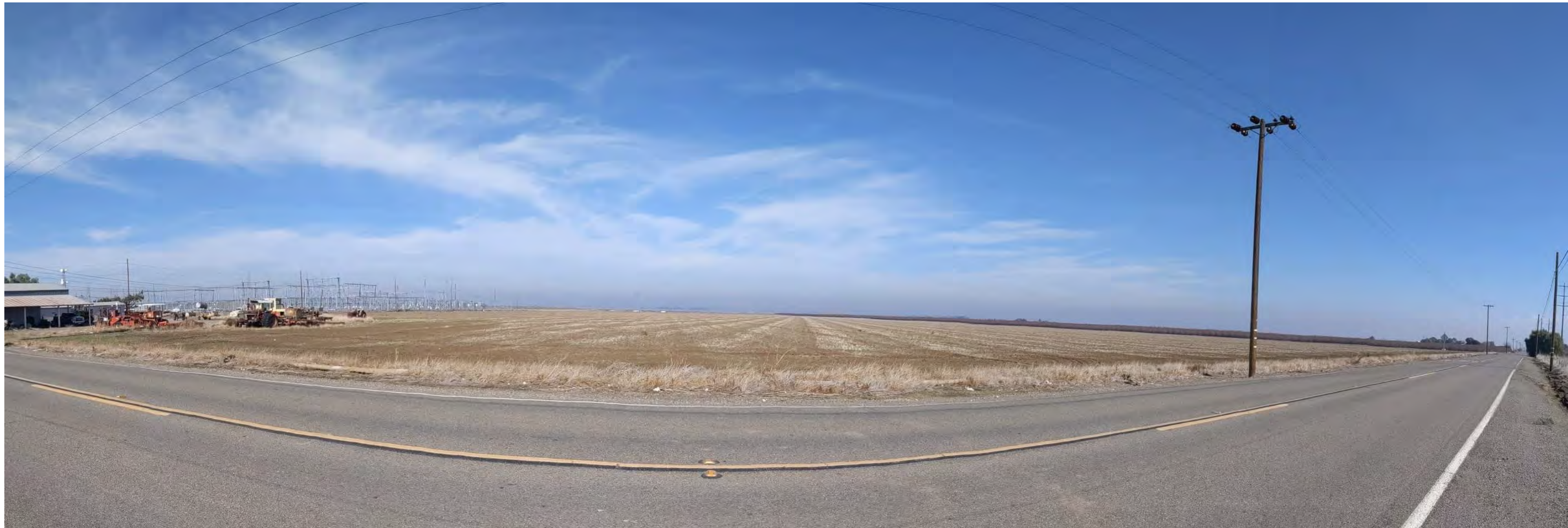
Photo taken from Kelso Road looking north
