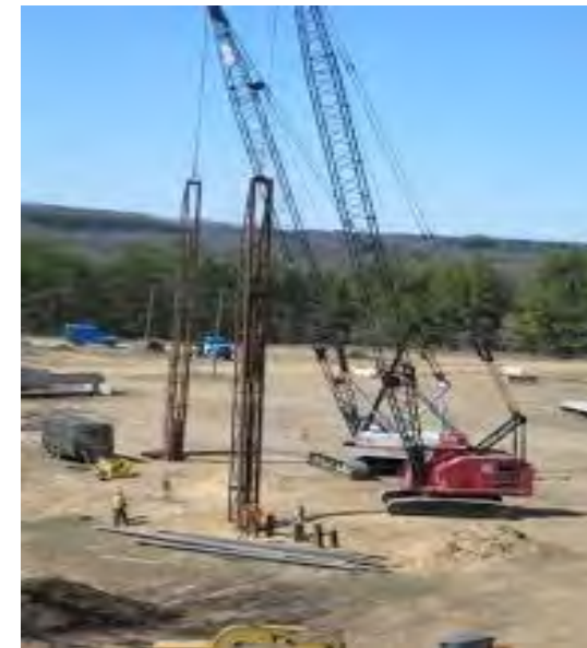
Pile Driver without Noise Reduction Equipment Source: Carpenters Training Institute
