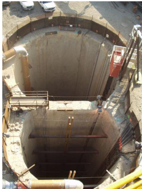
Figure 12. Double-cell Shaft Concept, Northeast Interceptor Sewer in Los Angeles
