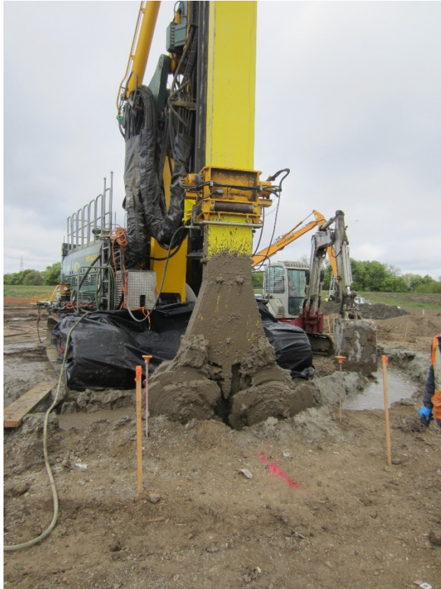
Figure 3. Deep Mechanical Mixing Rig with Cutters
