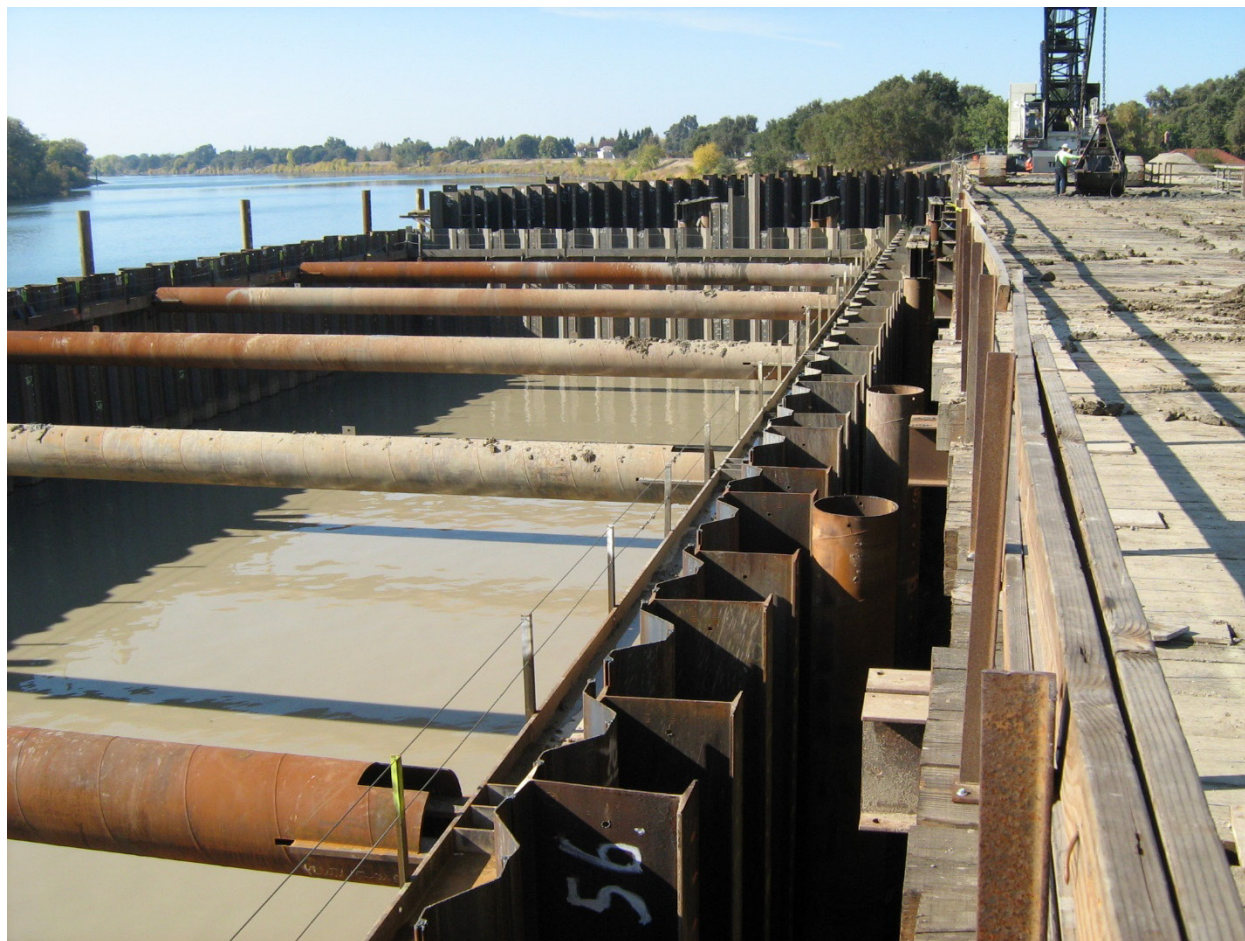
Figure 1. Cofferdam for Freeport Intake
