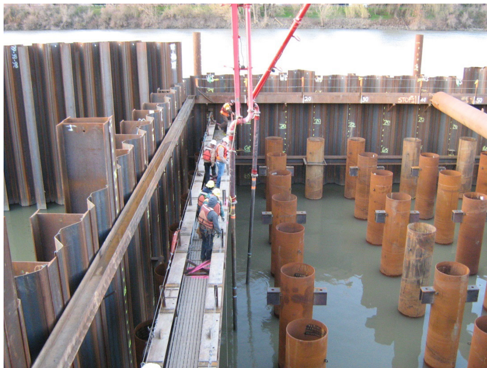
Figure 4. Tremie Concrete Placement at Freepoint Intake
